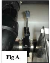
Macerator Cutoff Normal Position
