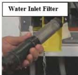
Draining the Aqua Go Water Heater
