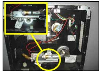
Fig 1: Water Heater Drain Plug
