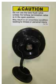
Tank Flush Inlet
