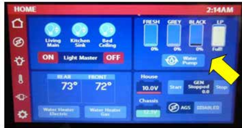
Touch Screen Tank Monitor example
