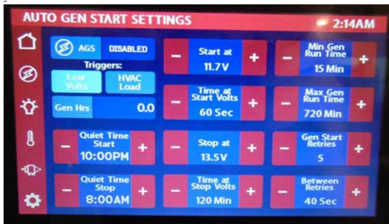
Example of a touch screen Generator settings
