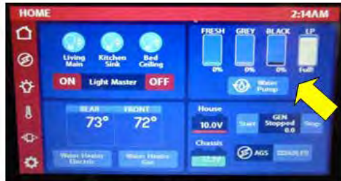
Touch Screen Tank Monitor example
