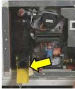
Draining the Aqua Go Water Heater
