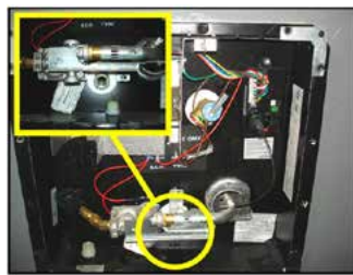
Water heater drain plug
